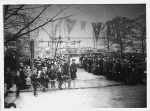
Laying of the foundation stone at Bitterne Park Congregational Church, 1905. William Jupe was present but cannot be identified. © Local Studies Collection, Civic Centre Library, Southampton
