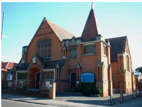
Bitterne Park Congregational Church, now United Reformed Church, Cobden Avenue
